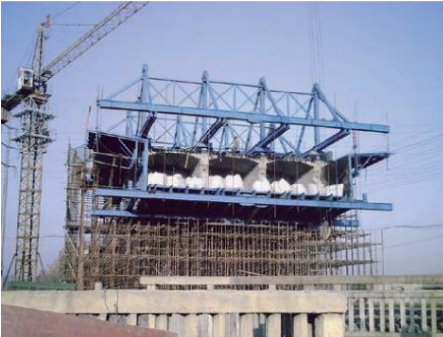
Construction site of Form Traveler for China Railway Tenth Group
